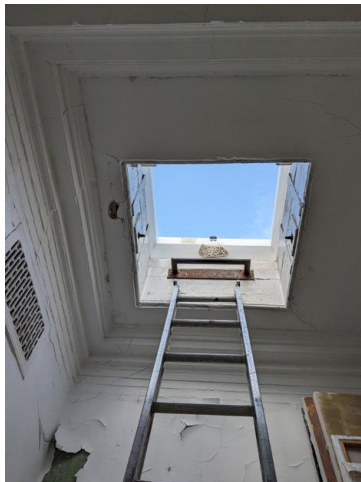
7.57 - Room 33 access hatch area
