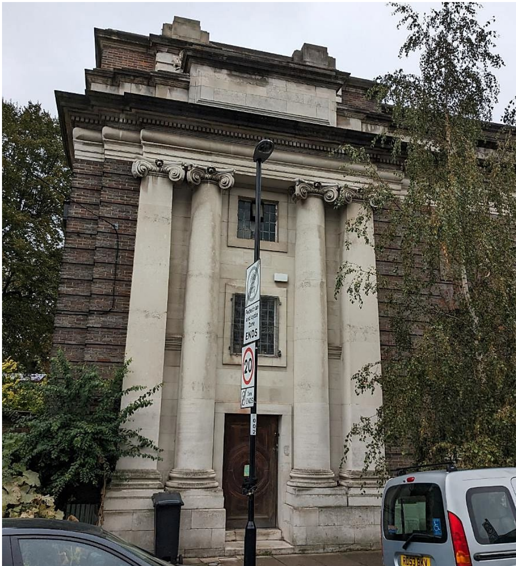
Fig. 4. South-east façade detail
