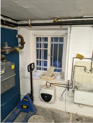
7.13 - Room 10 soffit and window
