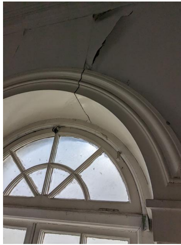
7.71 - Room 36 north-east edge
