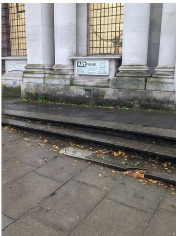
15.1 - Stone steps/ ramp at entrance
