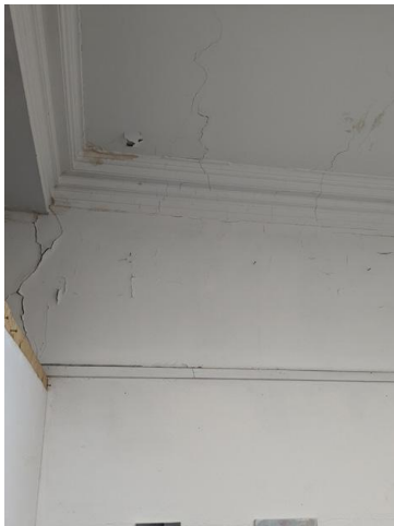
7.56 - Room 33 soffit and wall
