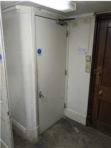
7.29 - Room 28 walls, doors, floors
