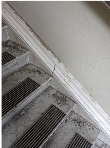
7.47 - Room 32 stair and skirting
