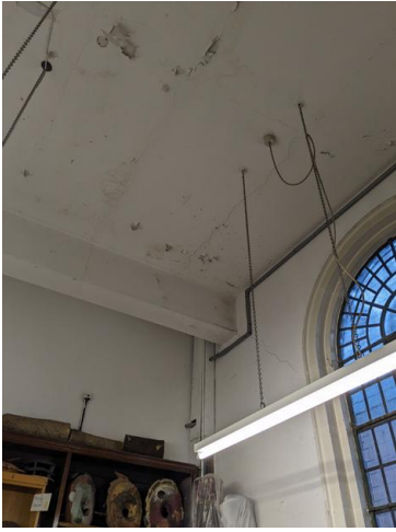
7.34 - Room 30 walls, soffit, downstand
