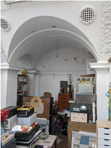
7.61 - Room 34 side vaults
