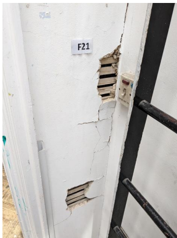
7.68 - Room 35 walls by room 36
