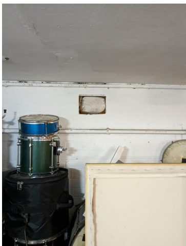
7.8 - Room 9 wall opening and soffit
