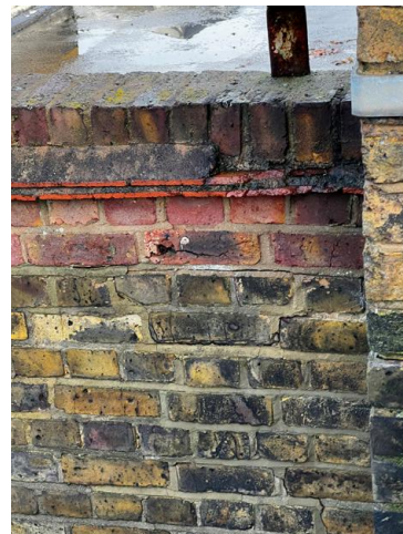
5.5 - Old scaffold tube fixing
