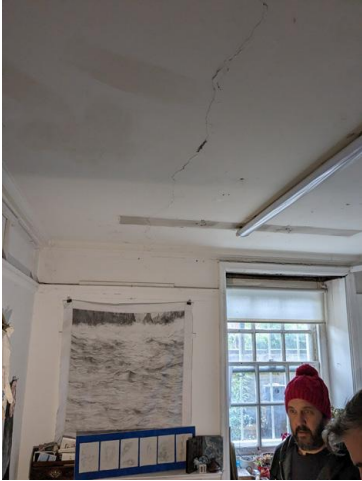
7.16 - Room 21 window and soffit
