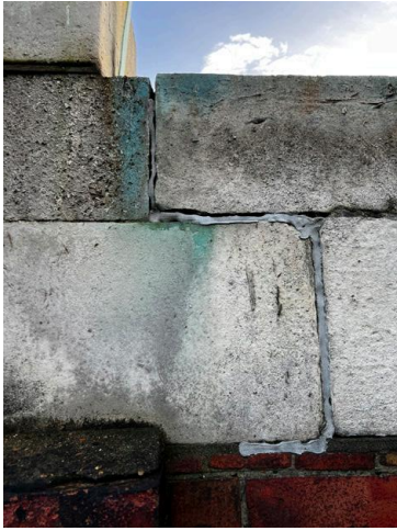
3.12 - Mastic filled joints
