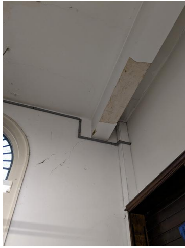
7.35 - Room 30 walls, soffit, downstand
