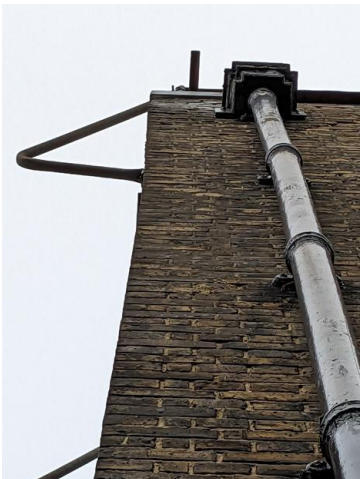
5.6 - West corner of staircase wall
