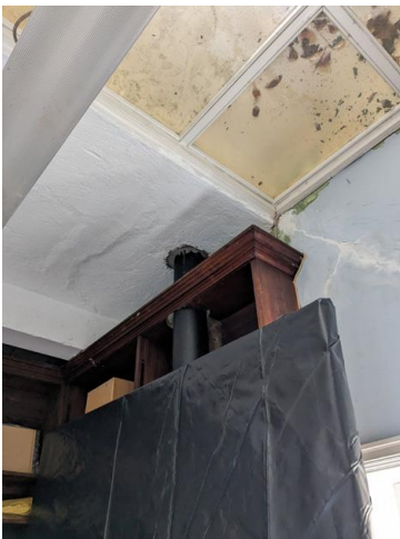
7.76 - Room 39 shelving and downpipe
