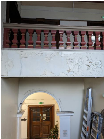
7.49 - Room 32 fascia and walls
