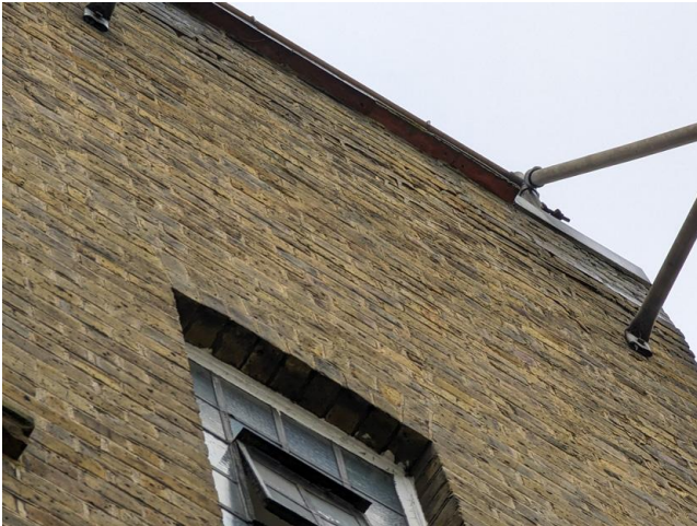
5.1 - SW facet of staircase wall
