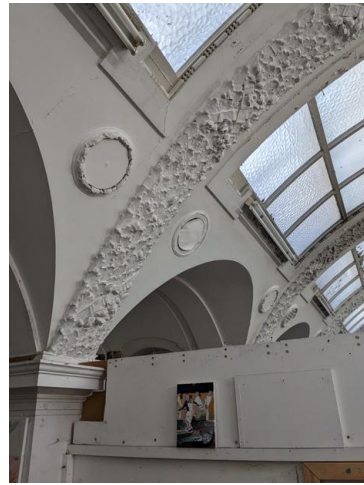
7.60 - Room 34 ventilation grilles
