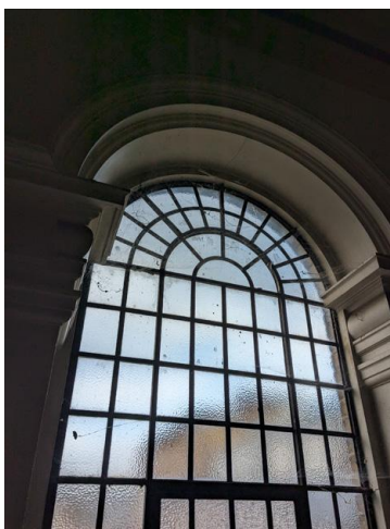
6.3 - Glazing in room 32 (staircase)
