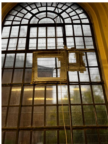
6.1 - Glazing in room 30 (studio)
