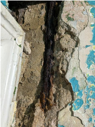
7.33 - Mezzanine WC wall
