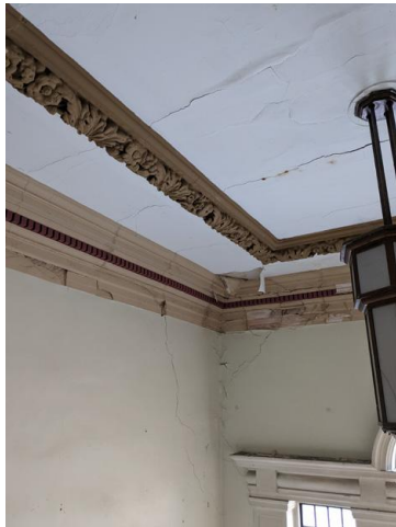
7.51 - Room 32 western corner
