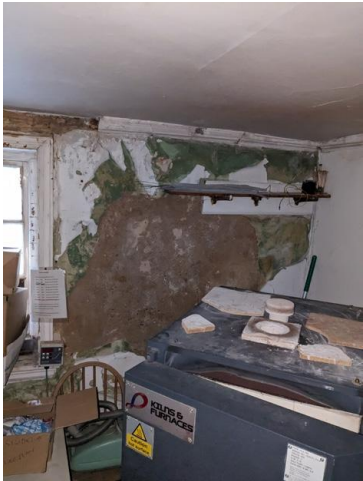
7.31 - Room 29 wall and window
