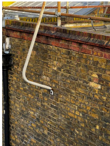
5.4 - Parapet jacking
