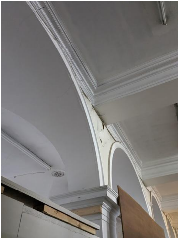
7.27 - Room 26 walls between arches
