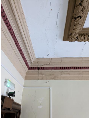
7.52 - Room 32 eastern corner
