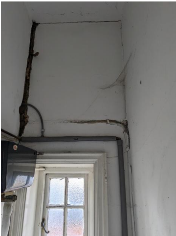
7.73 - Room 38 partitions and soffit
