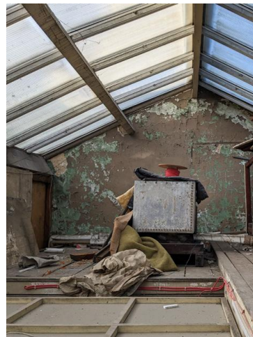
7.66 - Room 35 attic space
