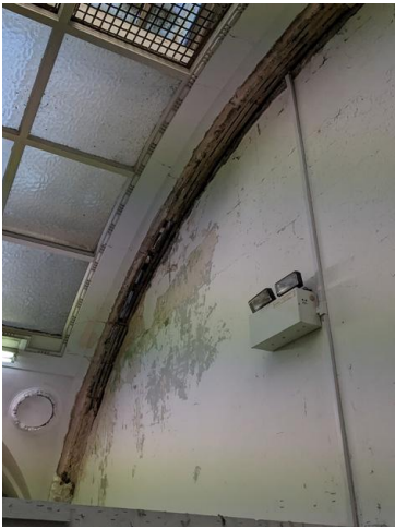
7.58 - Room 34 north-east end
