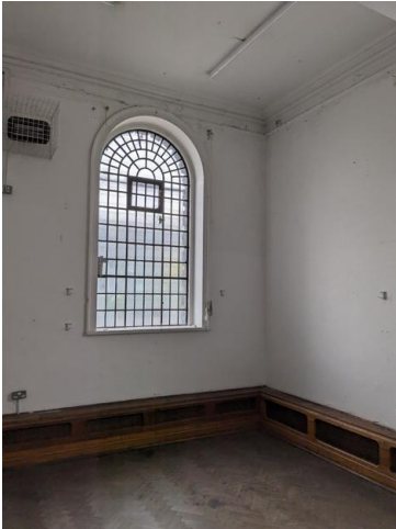
7.20 - Room 21 western corner
