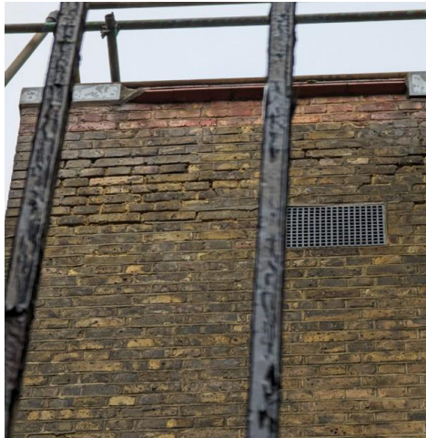
5.2 - SW facet of staircase wall
