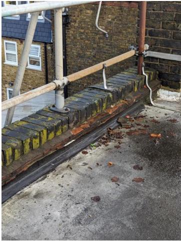
3.6 - Creasing tiles/ mortar fillet
