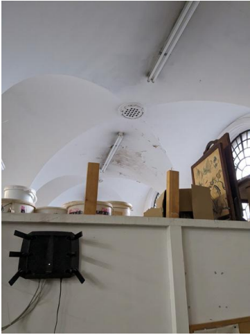
7.24 - Room 26 vaulted ceiling
