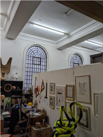
7.26 - Room 26 soffit and downstands
