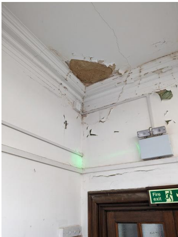
7.55 - Room 33 southern corner
