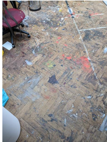
7.42 - first floor parquet flooring
