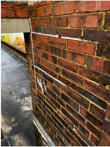
3.11 - Mastic filled joints
