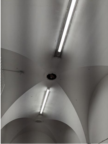
7.18 - Room 20 vaulted ceiling
