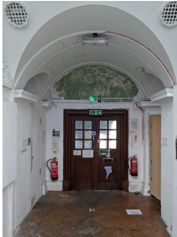
7.62 - Room 34 door to staircase
