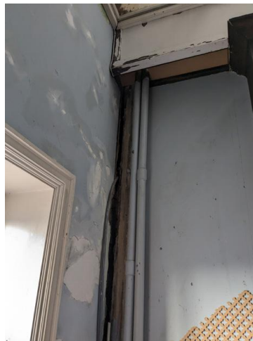
7.77 - Room 39 walls and partition
