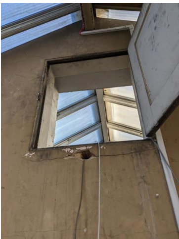
7.67 - Room 35 hatch in attic space
