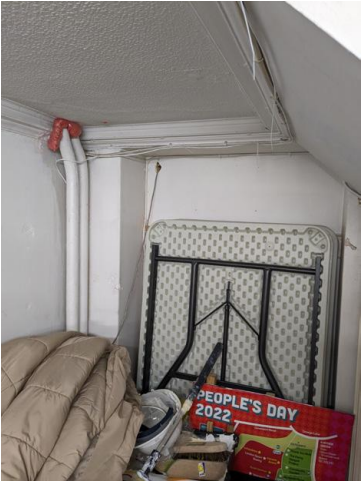
7.37 - Room 31 walls and services
