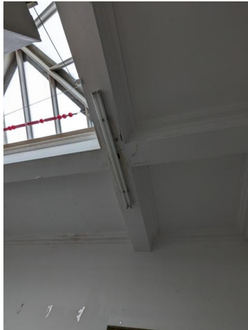
7.54 - Room 33 soffit and downstands
