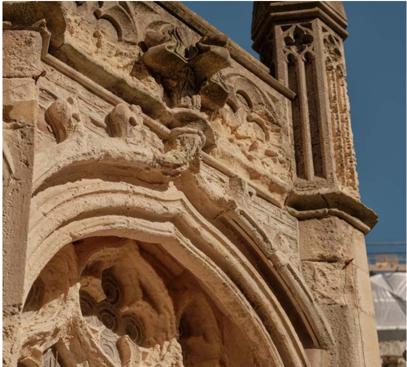
Crumbling stonework before restoration
